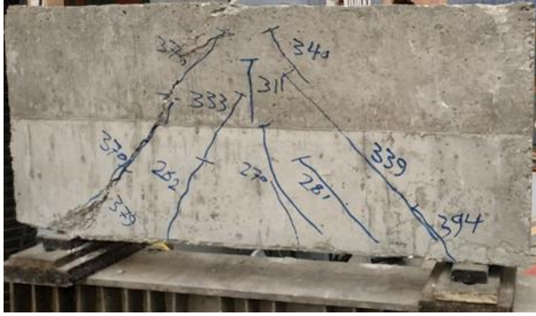
B1: Shear failure
